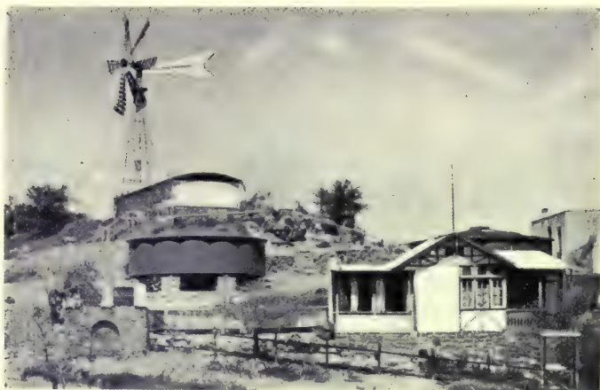
THE WATERWORKS, WINDHOEK.
